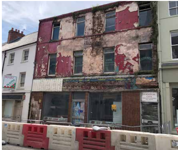
Dilapidated building, Bridge Street
